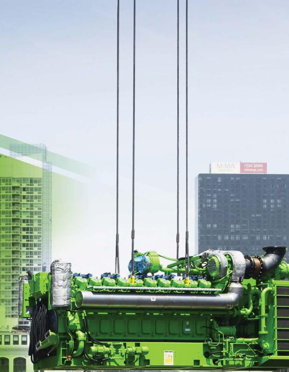
One of four Jenbacher J620 gas engines being lifted by crane into place for the Hudson Yards project in New York City. Photo courtesy: GE
